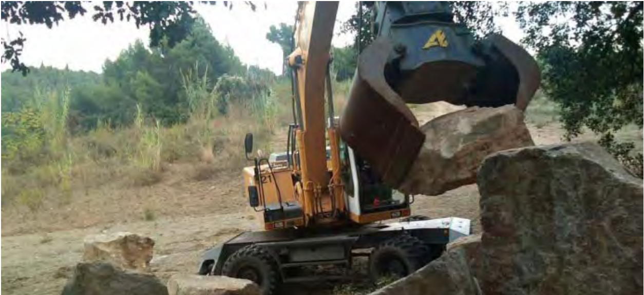
DIGGER WITH HYDRAUIC CLAMP MOVING ROCK
