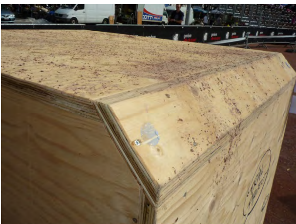
Avoid corners in 90° on impact areas to avoid damages on the structure
