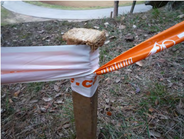
Fig. 2: Fix the tape by winding it round the stakes twice; ensure the tape is secure
