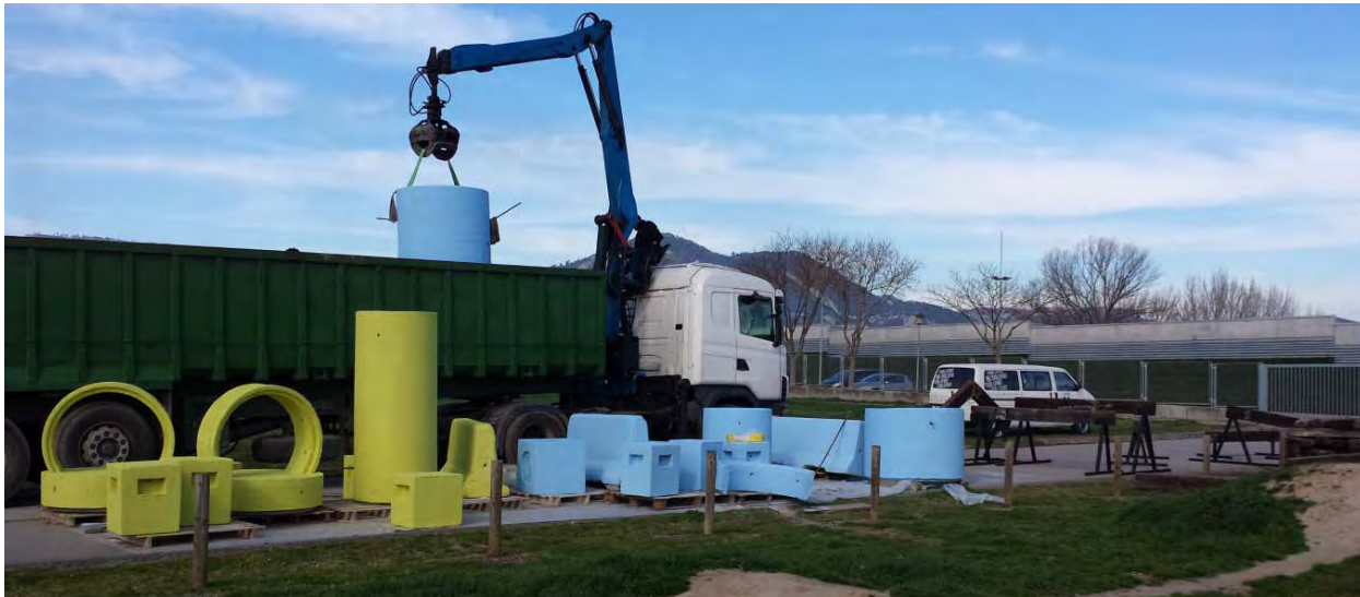
LORRY WITH A CRANE MOVING PRECAST CONCRETE PIPES
