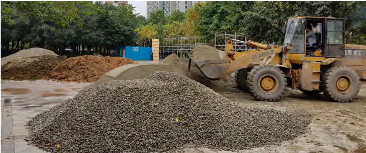
LOADER SPREADING GRAVEL AND POWDER STONE
