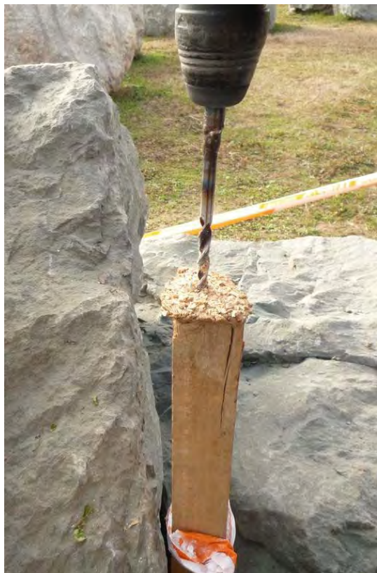
Drill into the wooden stake
