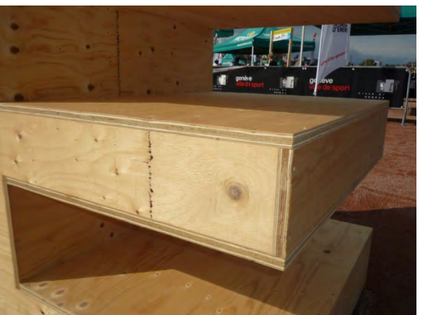
Avoid corners in 90° on impact areas to avoid damages on the structure
