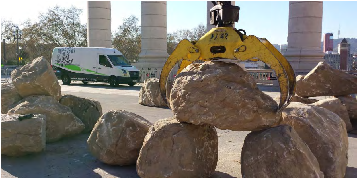
DIGGER WITH HYDRAUIC CLAMP MOVING ROCK
